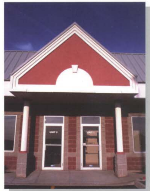
COMMERCIAL BLDG. 25 STRUCT CRT. CAMBRIDGE, ONT.
